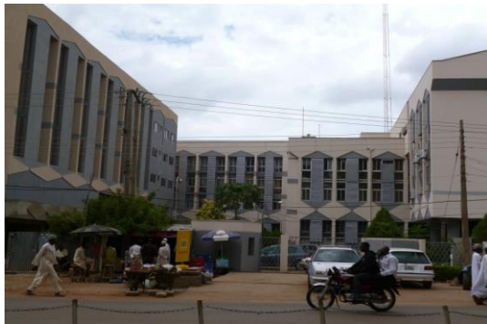
National Board for Technical Education Headquarters (1988)
